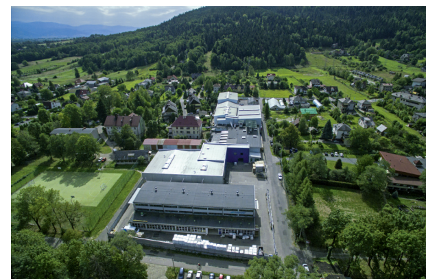
Buczkowice – production & warehouse
